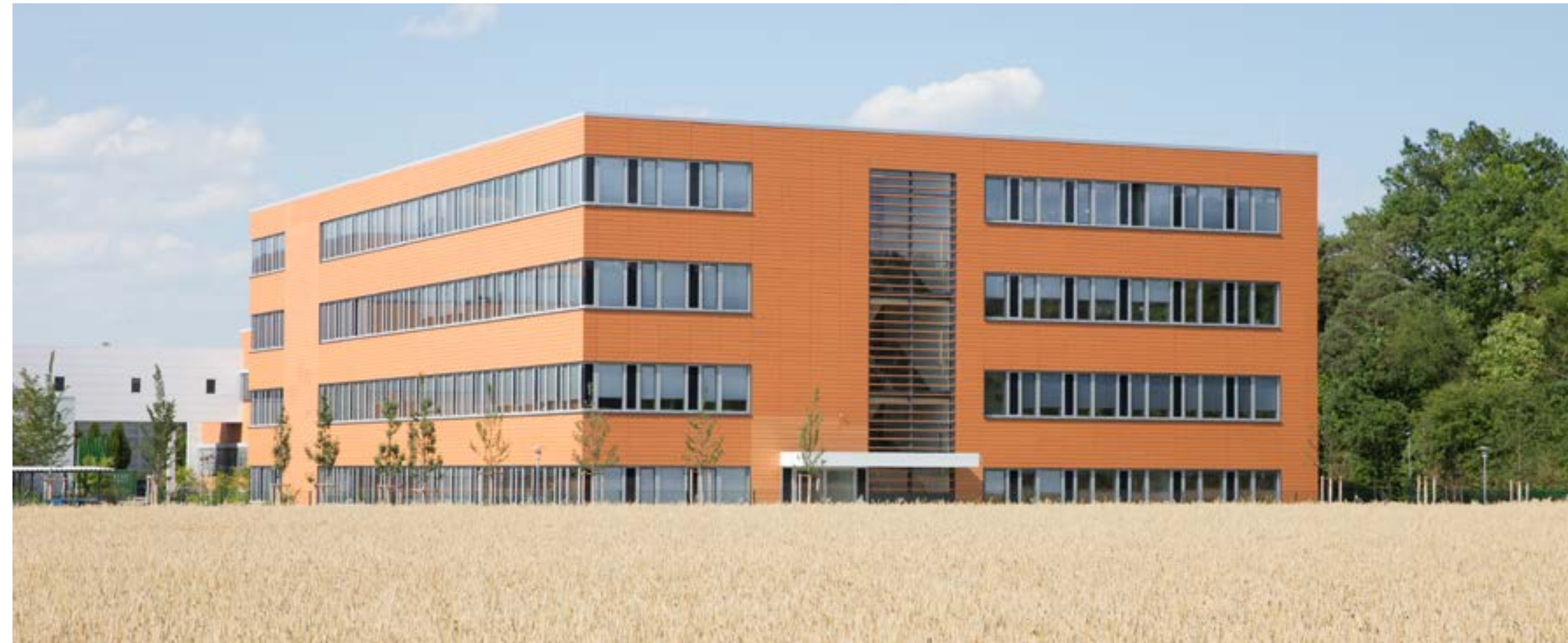
Green building at company headquarters in Oberschleissheim
